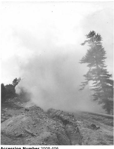
Blast breaking up a granite bed in the path of the oil pipeline. From the scrapbook War Emergency Pipelines, Inc.: Construction Views - First Section of East Texas-East Coast Pipeline.
