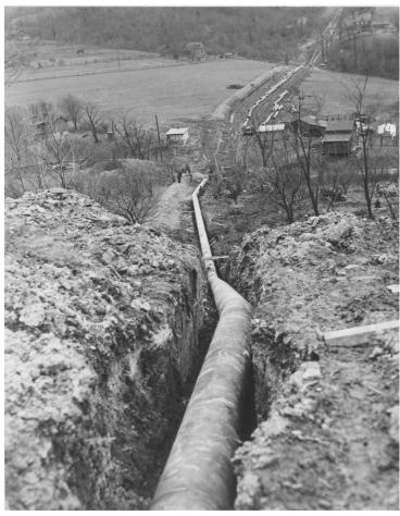
Section of oil pipeline with overbends and side bends as it enters the Western slopes of the Alleghenies in Western Pennsylvania. The combination bend was factory-made by the National Tube at Lorain. From the Scrapbook War Emergency Pipelines, Inc.: Construction Views, Eastern Extension of East Texas-East Coast Pipeline, Volume I.
