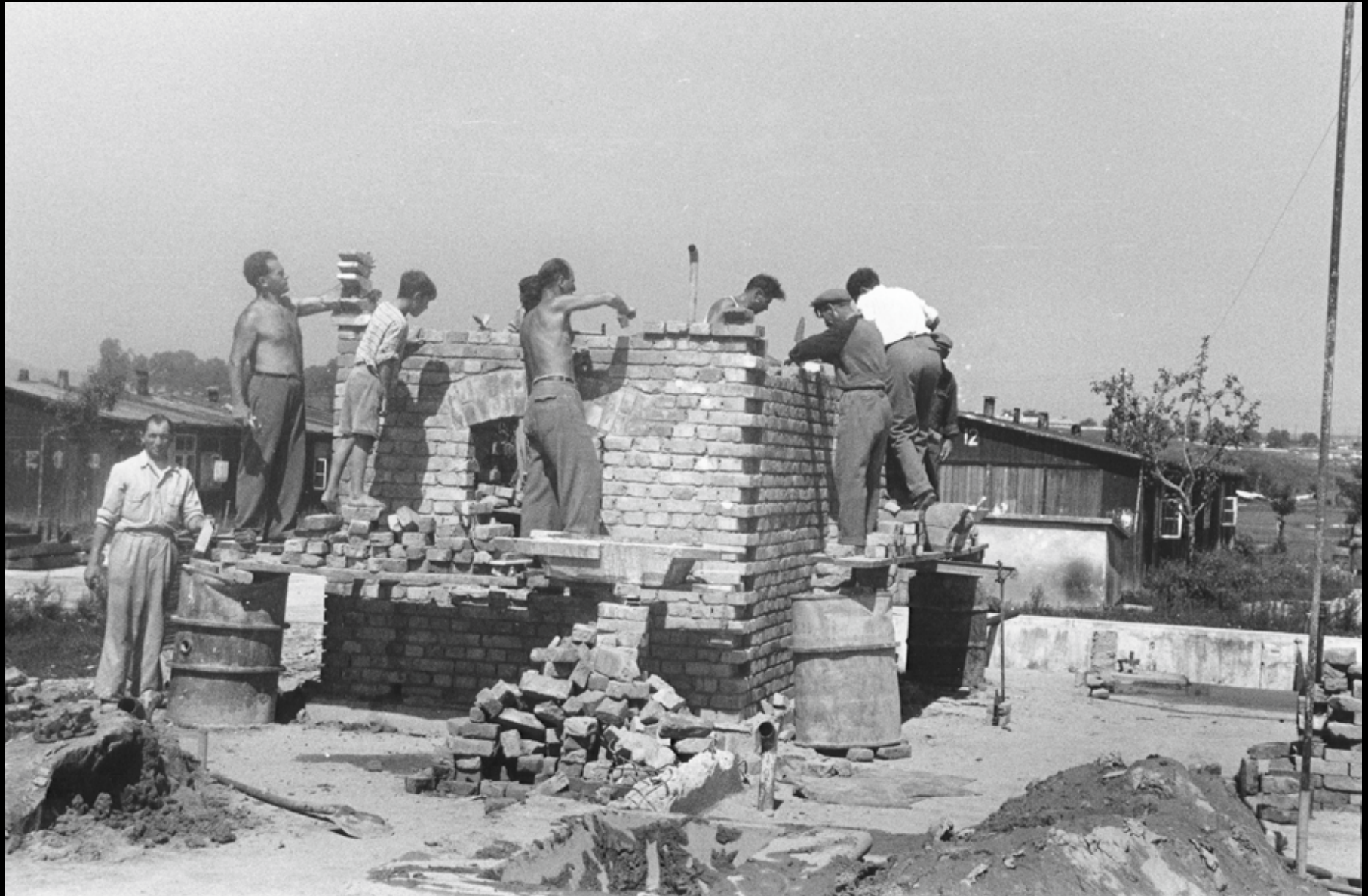
Under the guidance of an ORT instructor, Jewish DPs learn bricklaying by constructing a small brick building at a Jewish displaced persons camp in Linz.
